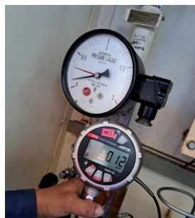
Gambar 8. Pengujian Differential Pressure Indikator
