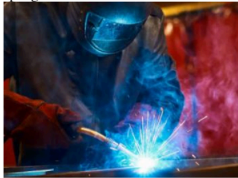
Gambar 4. Proses Pengelasan Metal Inert Gas (MIG)
