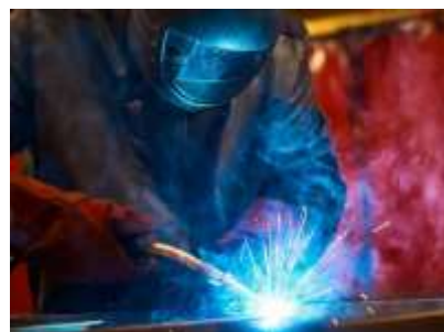
Gambar 4. Proses Pengelasan Metal Inert Gas (MIG)
