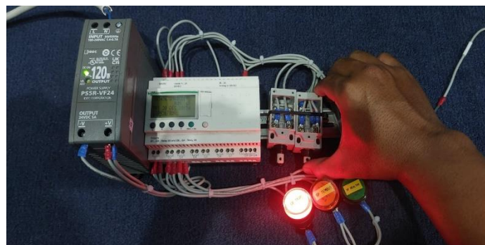
Gambar 14. Kondisi Sudden Pressure Trip
