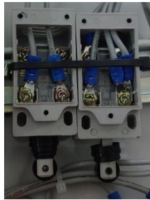
Gambar 4. Switch Terminal Sudden Pressure
