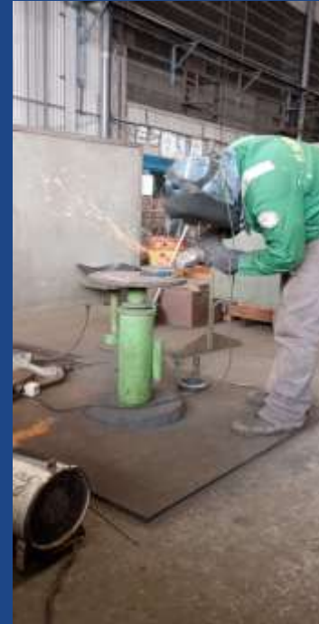
Proses fit-up pipa
